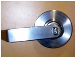
**TYPE 3. Square slot hidden behind metal cap.** Remove cap with fingers. Then use square override key provided by PO&M (image below). Put key in slot and turn.
